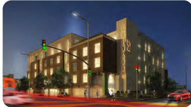
5144 CRENSHAW | LOS ANGELES, CA MULTIFAMILY | 79 UNITS UNDER CONSTRUCTION
