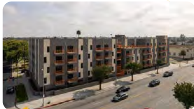
1650 W FLORENCE AVE | LOS ANGELES, CA MULTIFAMILY | 128 UNITS DELIVERED 2022
